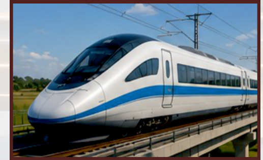
Ahmedabad Dholera Semi High Speed Rail
